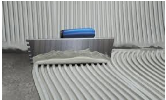
Use the Notch sized to control adhesive application as needed.
