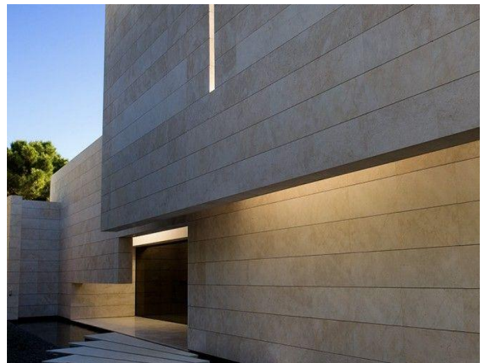
BS Tileasy 400 used for Large Stone tiles application on Facade Wall.
