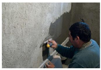
Application of BS Tileasy-F on Wall over smooth levelled / plastered surface.
